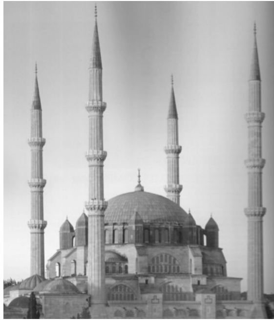
Fig. 8.8 The Selimiye Mosque with its large central dome flanked by four minarets. Sinan identifies the dome with the Prophet and the four minarets to the “Rightly Guided Caliphs” (Source: Kuban 2010, 296)
