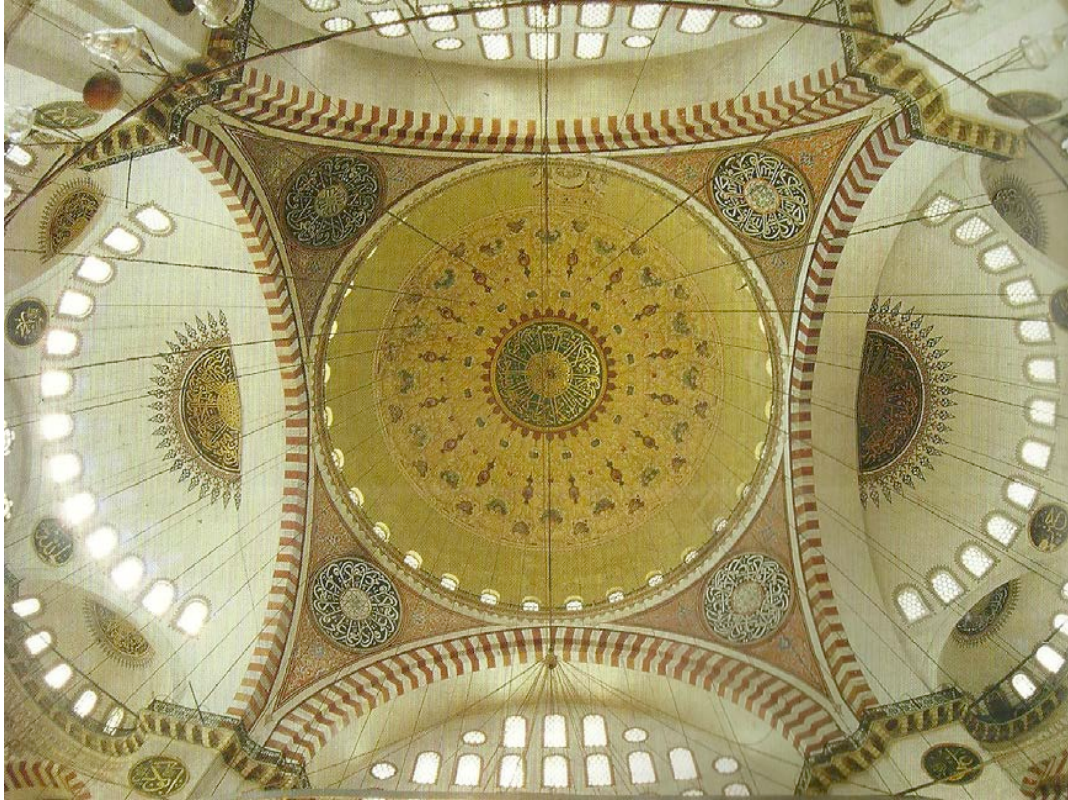
Fig. 8.7 Interior view of the Süleymaniye mosque main dome supported by four columns and arches. (Source: Necipoğlu 2011, 215)
